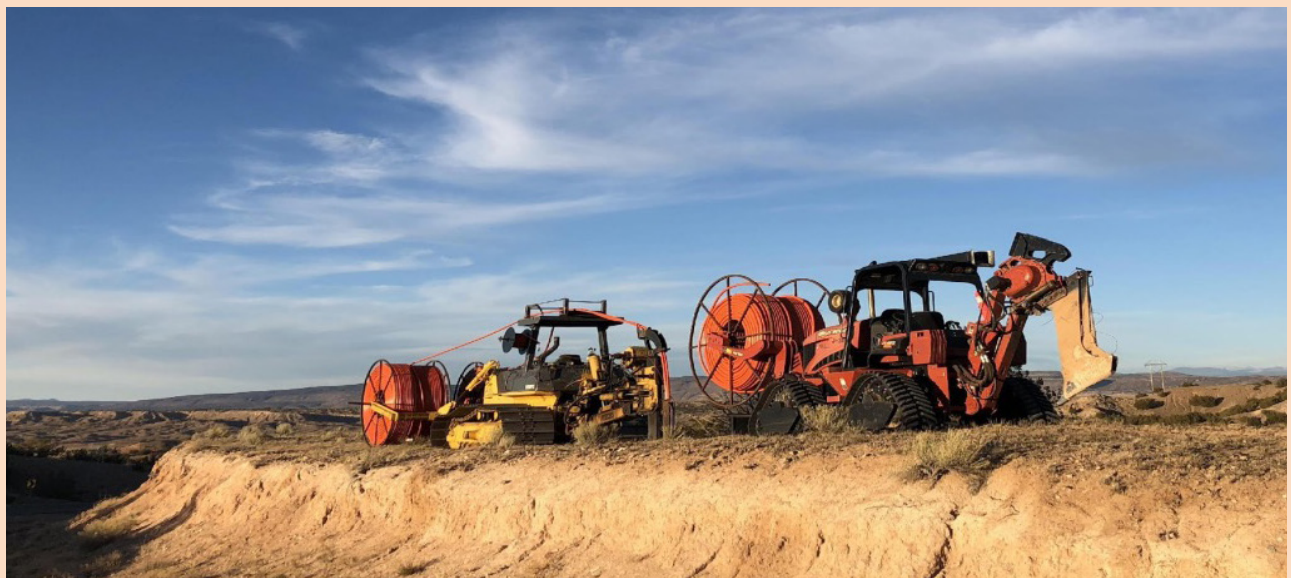
Ploughs are able to 'sew' the conduit into the ground by cutting a 6" opening to lay the conduit at depth without the labor costs and invasiveness of a backhoe to complete the same job.
