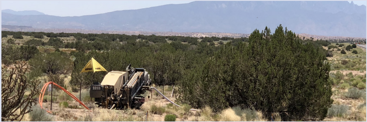
Kelly Cable of NM Directional drilling equipment utilizes trenchless technology on the Jemez-Zia project to install the conduit for the fiber optic cable across rugged terrain, such as arroyos, or under roads.
